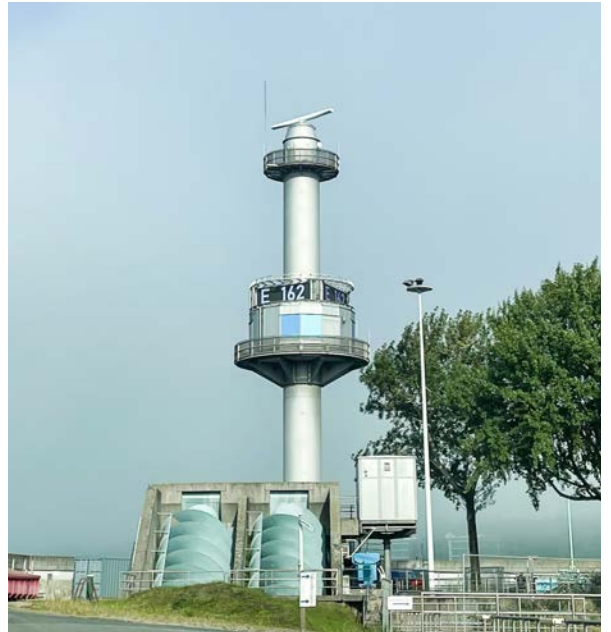
Water level indicator | Hamburg harbour
